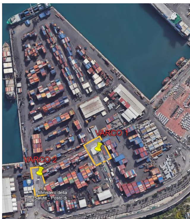
Figura 1 - Area SCT Terminal
